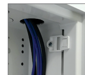
Installed SMC for affixing sidewall to stud.
